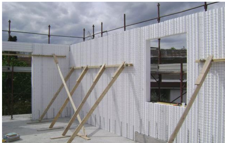
Figure B2 – Alignment operations of panels.
